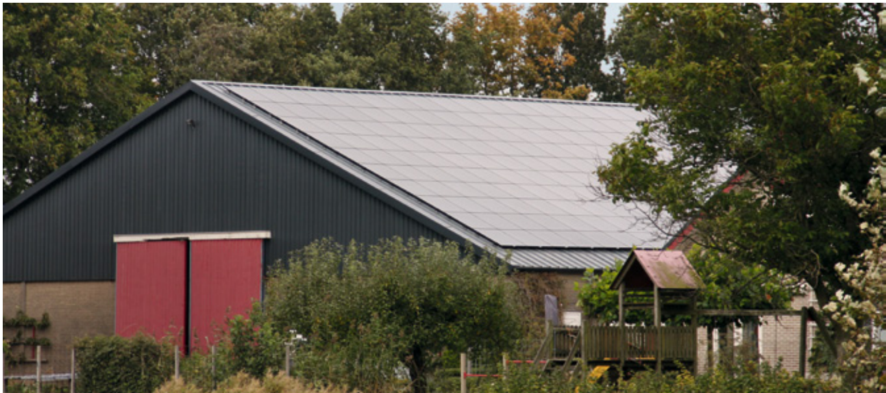
The black color of the Solar Frontier thin-film modules fit in perfectly with the new black cladding of the barn rooftop. (Image: SolarClarity)
